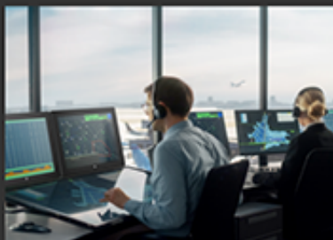
Air Traffic Control System
